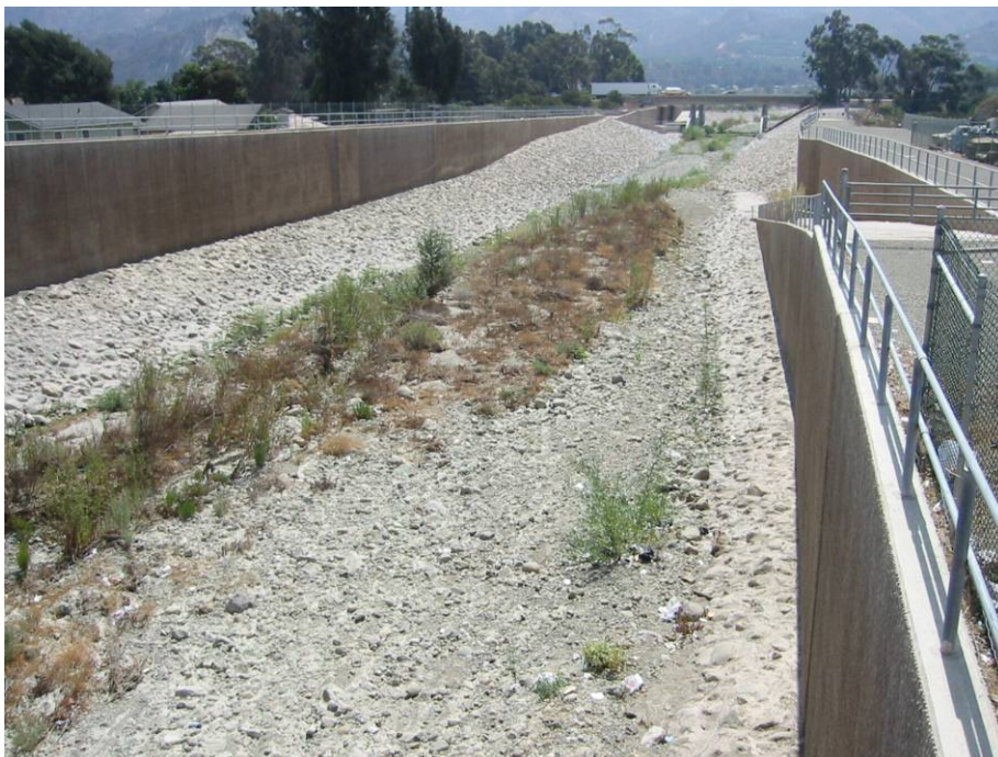
Figure 3-19. Looking downstream at Telegraph Avenue bridge.
