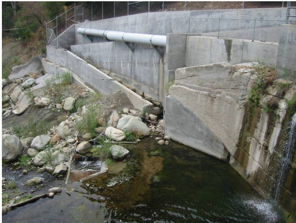
Figure 3-21. Looking downstream at Harvey Diversion Dam fish ladder.
