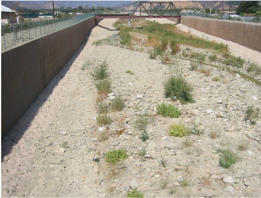
Figure 3-18. Looking downstream at the Southern Pacific Transportation Company (SPTC) truss bridge.
