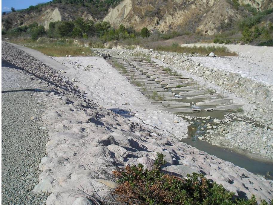
Figure 3-22. Looking upstream at US Army Corp of Engineers (USACOE) fish ladder.
