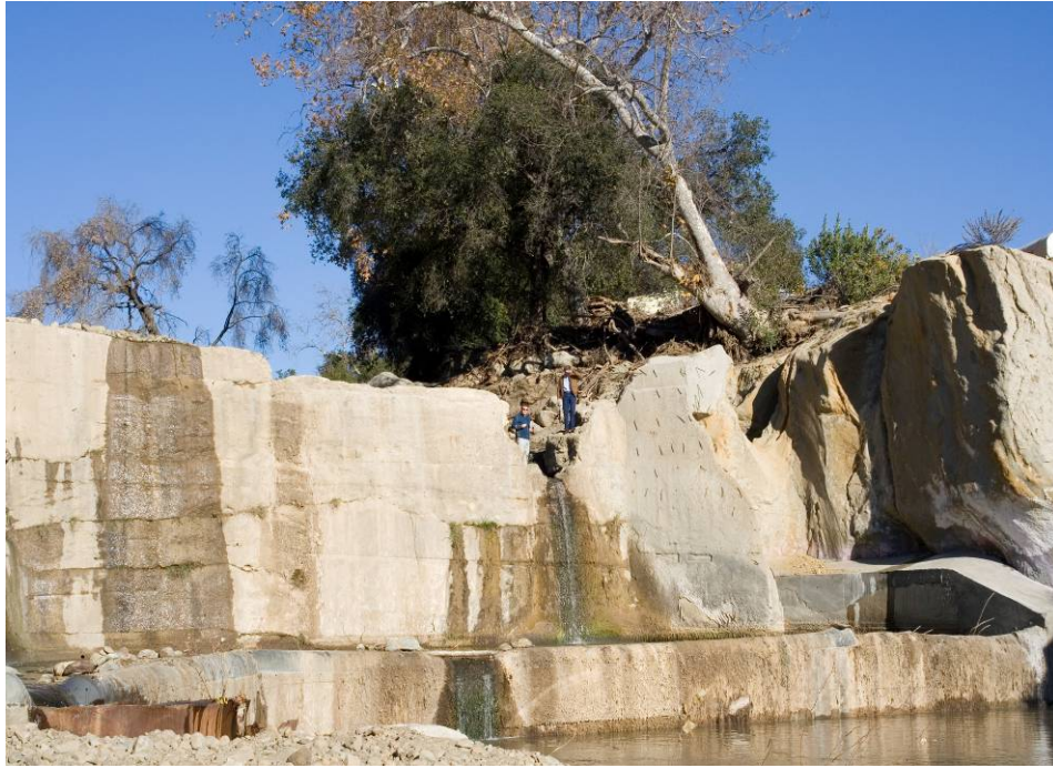
Figure 3-20. Looking upstream at damage to Harvey Diversion Dam following 2005 storm event.
