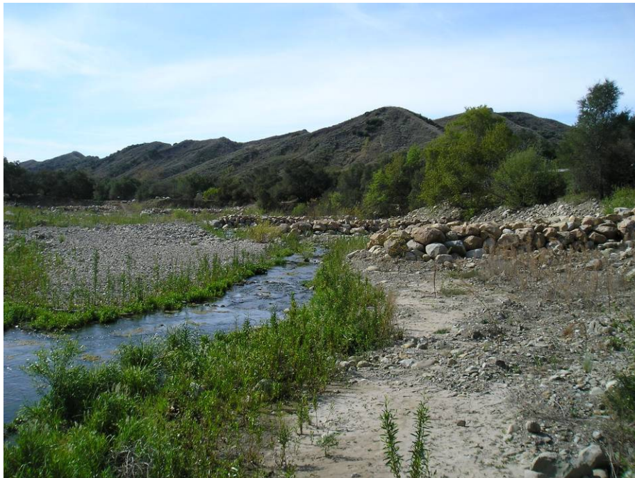
Figure 3-23. Looking downstream at right bank spur dikes in R4.
