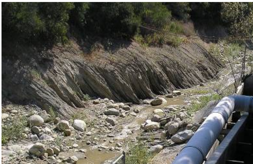
Figure 2-18. Recent scour of Santa Paula Creek associated with bedload-transport-restricting structures and presumably expressing an imbalance between transport capacity and sediment supply (a) below the lower Highway 150 crossing; and (b) below the Harvey Diversion Dam.
