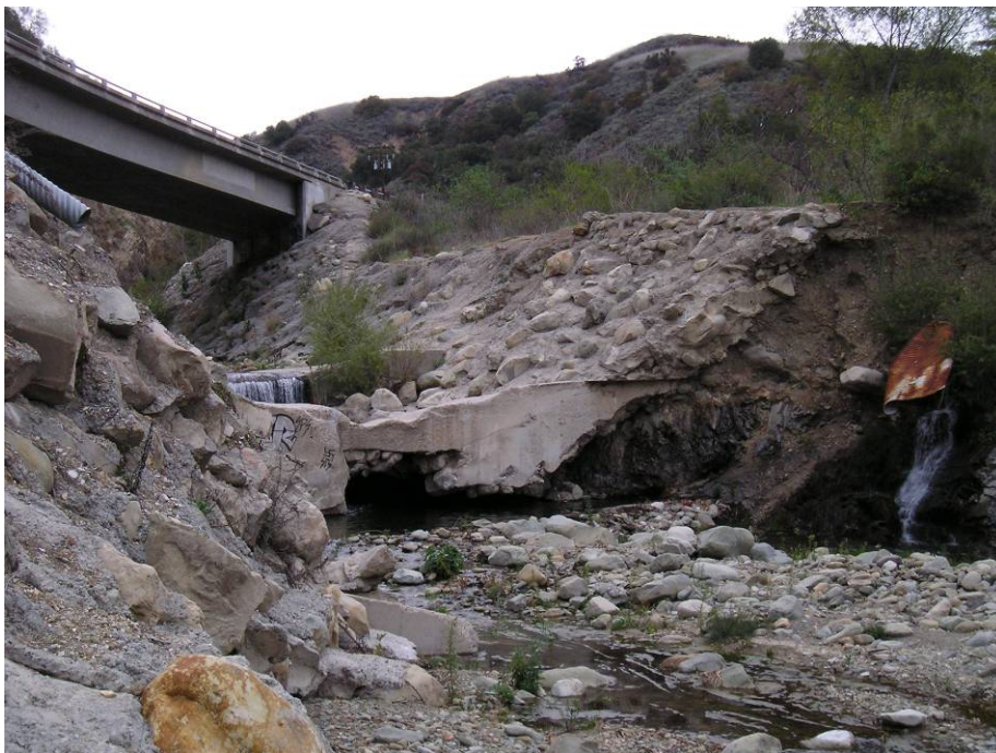
Figure 3-17. Looking upstream at Highway 150 grade control structure and channel incision.
