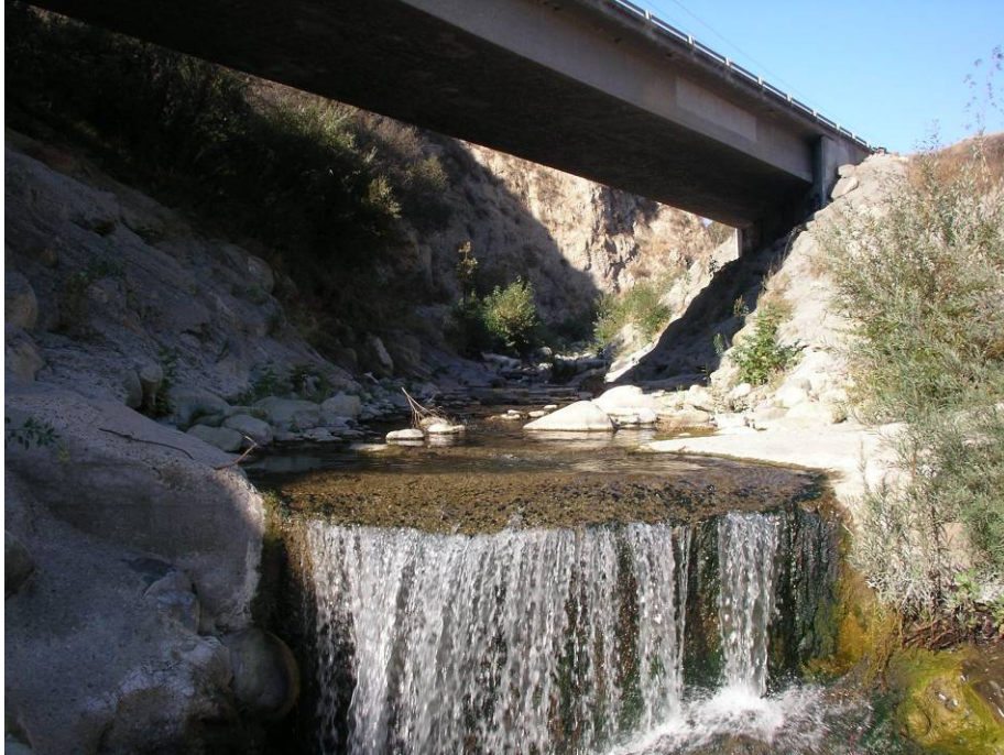
Figure 3-16. Looking upstream at Highway 150 bridge.
