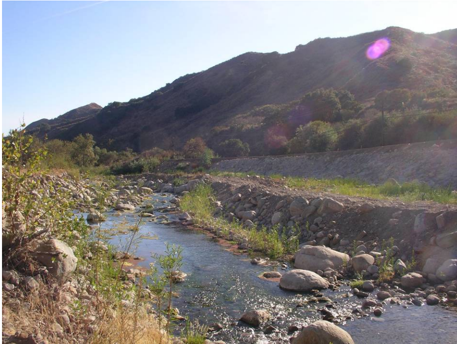
Figure 3-24. Looking downstream at channel realignment in R5.
